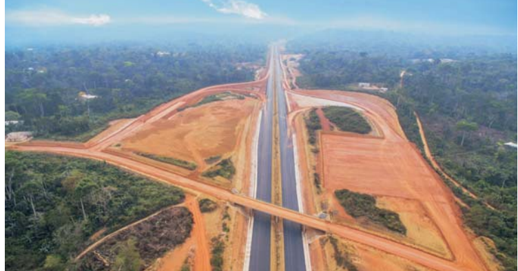
Autoroute Yaoundé – Douala (Cameroun)
